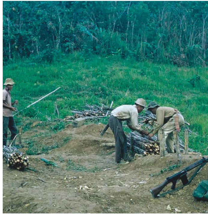
Labourers gathering timber for making a fascine.
